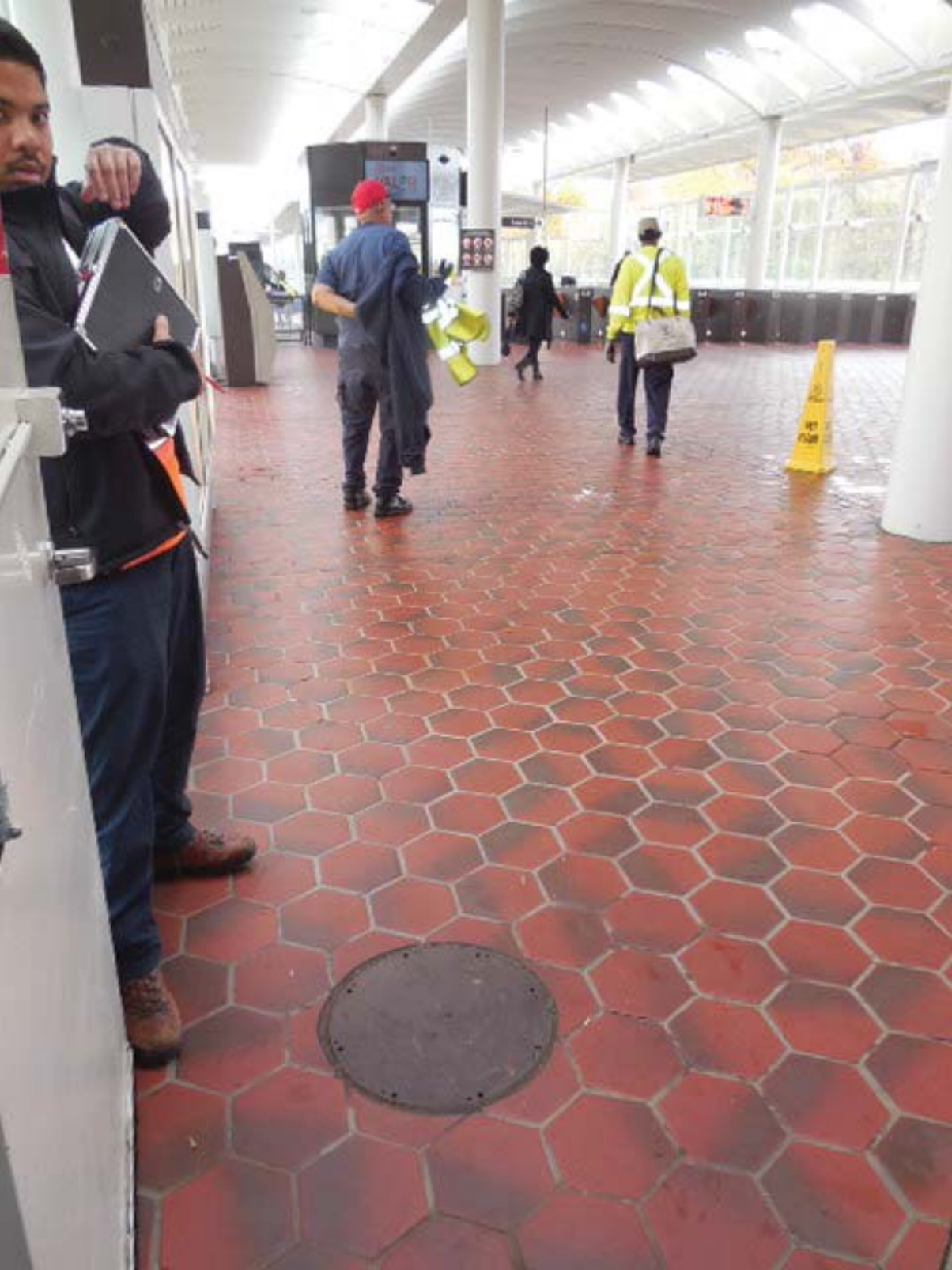
Picture 1: G04 Morgan Boulevard – Manhole in Mezzanine
