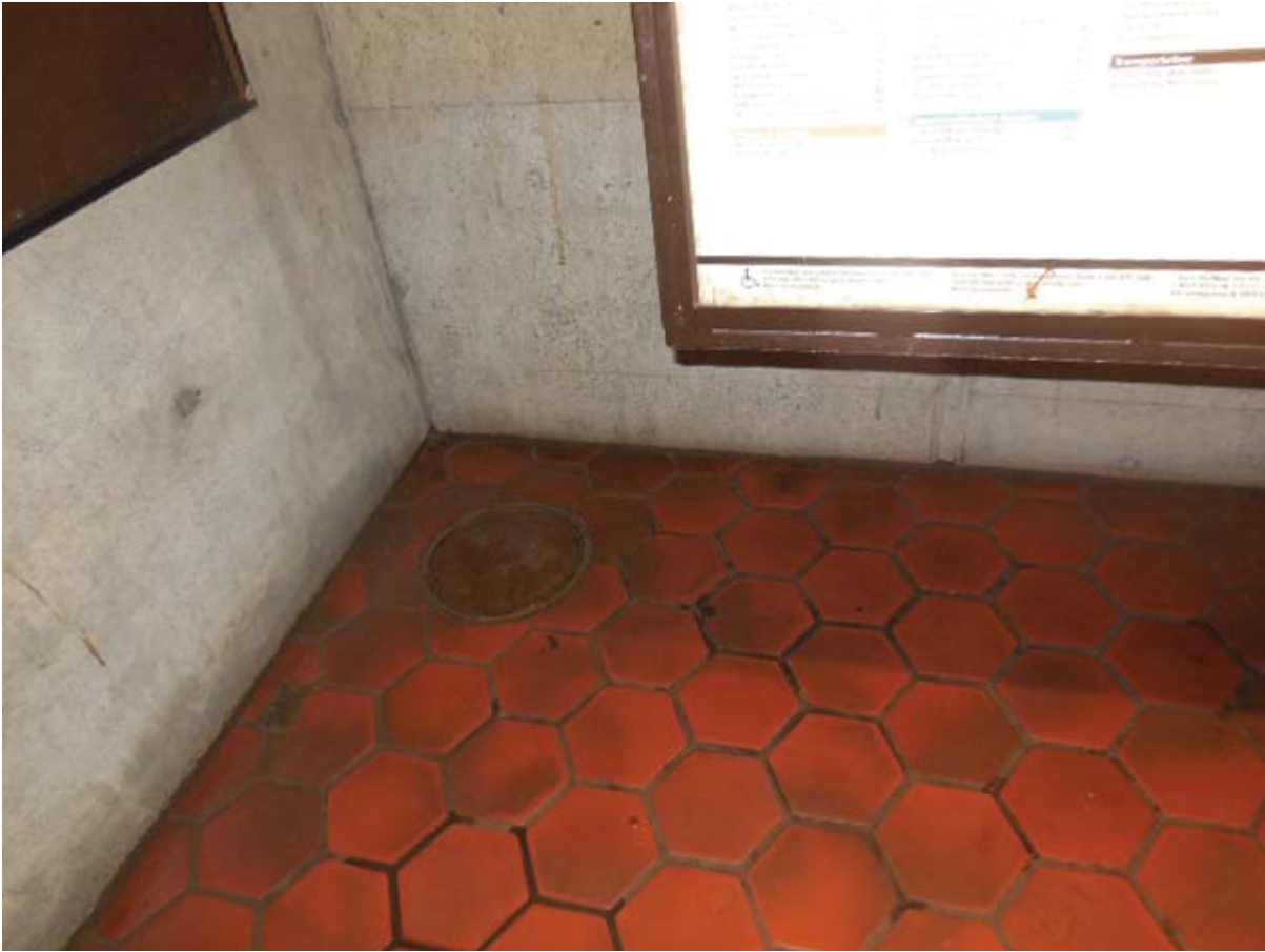
Picture 2: G01 Benning Road – Manhole in Mezzanine
