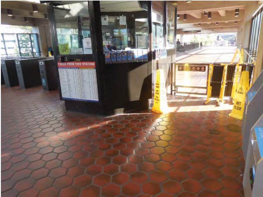
Photo #1: J03 Franconia-Springfield – Station Kiosk Area
