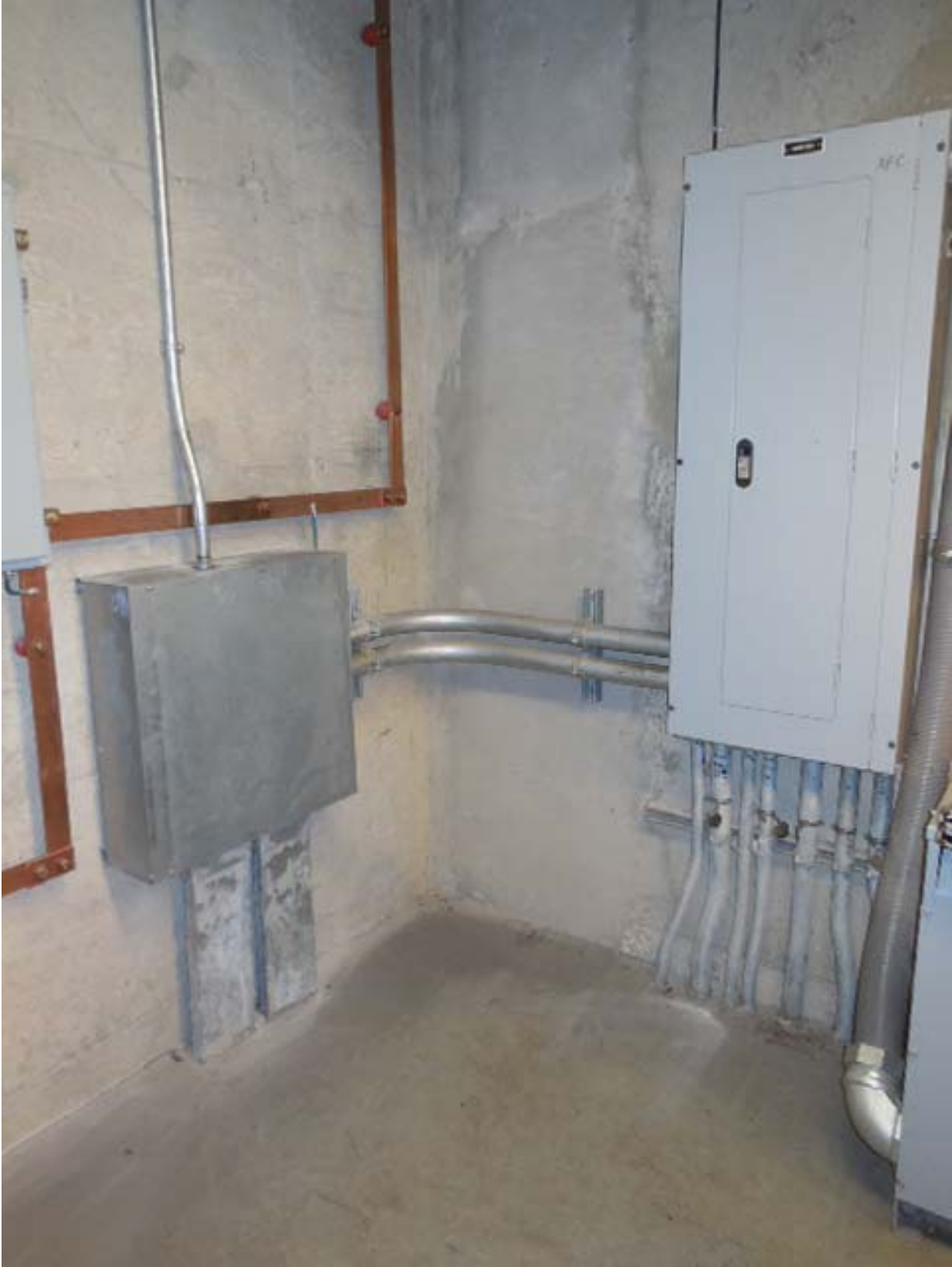
Picture 4: G04 Morgan Boulevard – AFC Panel WMESSI in Room 205
