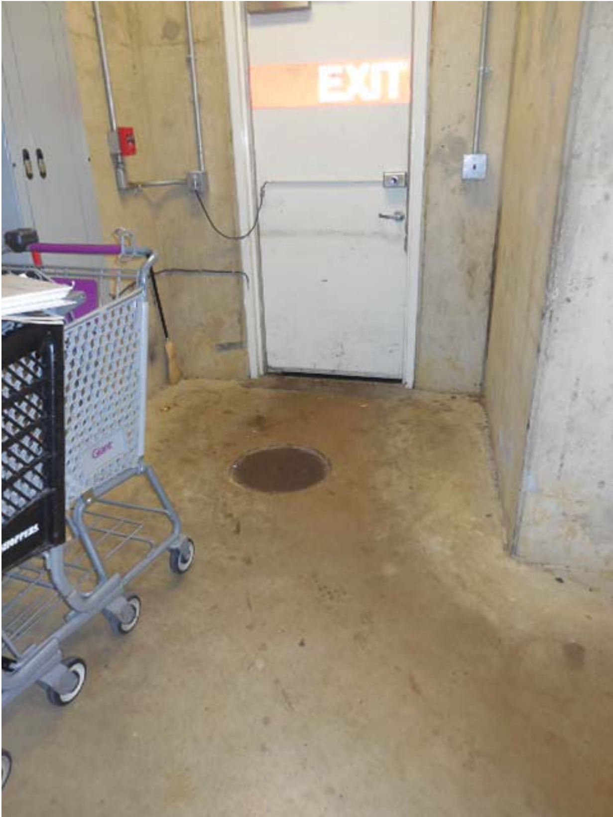
Picture 3: G05 Largo Town Center – Manhole in Service area
