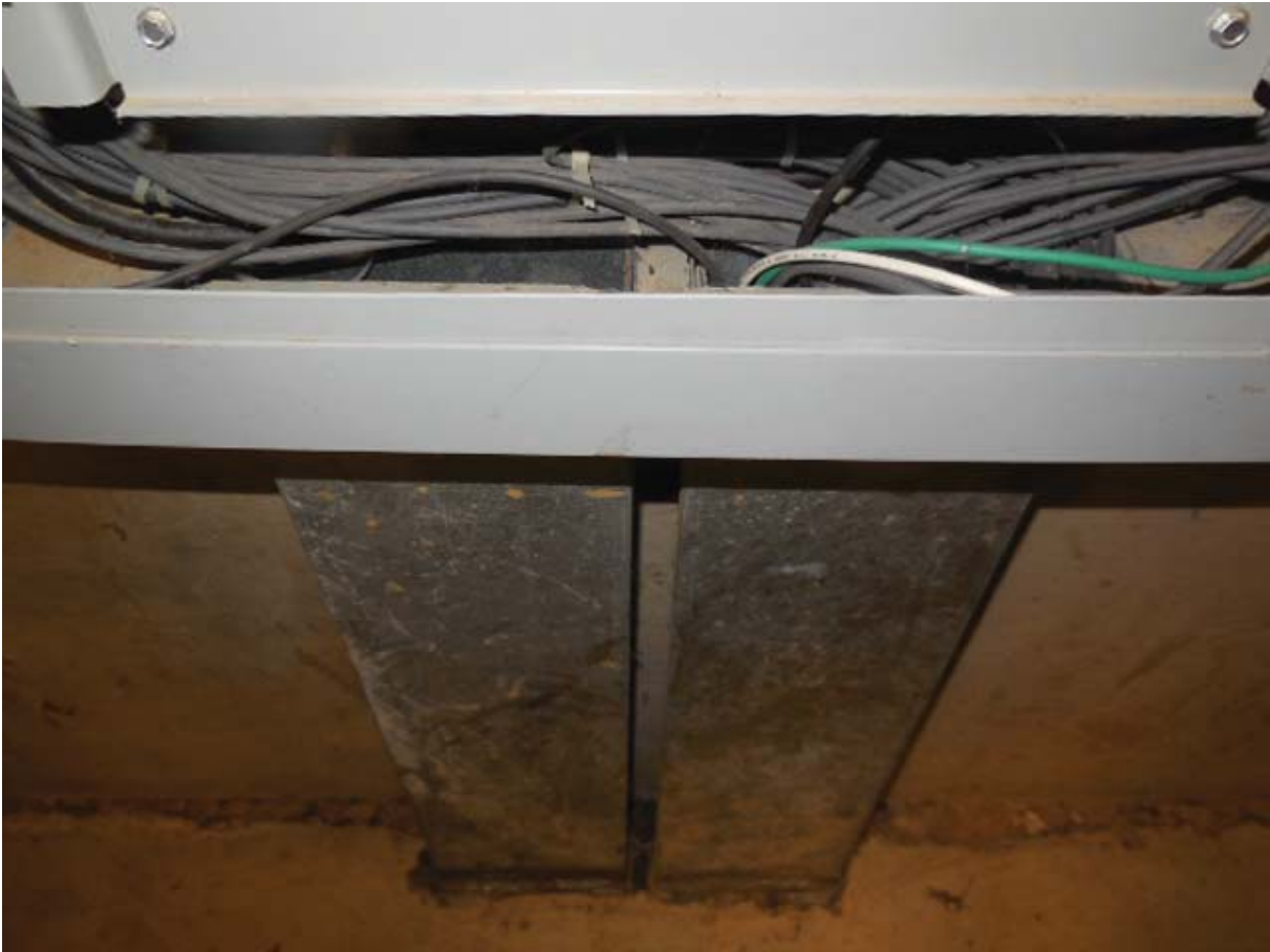
Picture 6: G05 Largo Town Center – AFC Panel WMESS1 in Room 117
