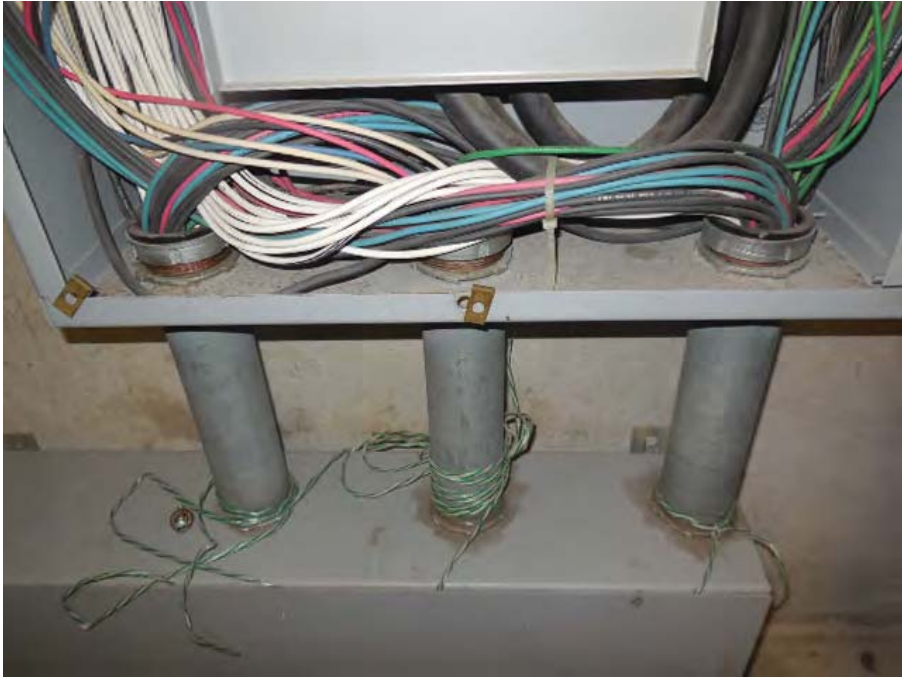
Photo #6: J03 Franconia-Springfield – Bottom of AFC Panel FF feeding into trough in Room 216
