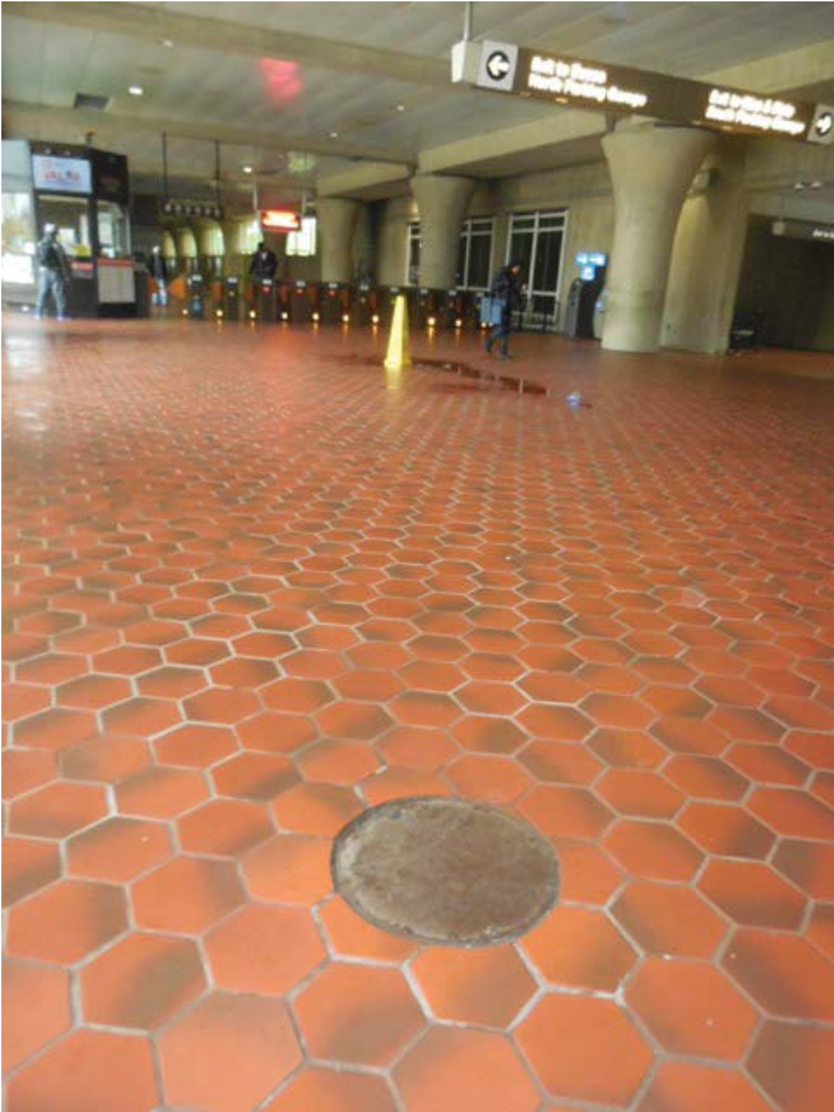
Picture 1: G05 Largo Town Center – Manhole in Mezzanine
