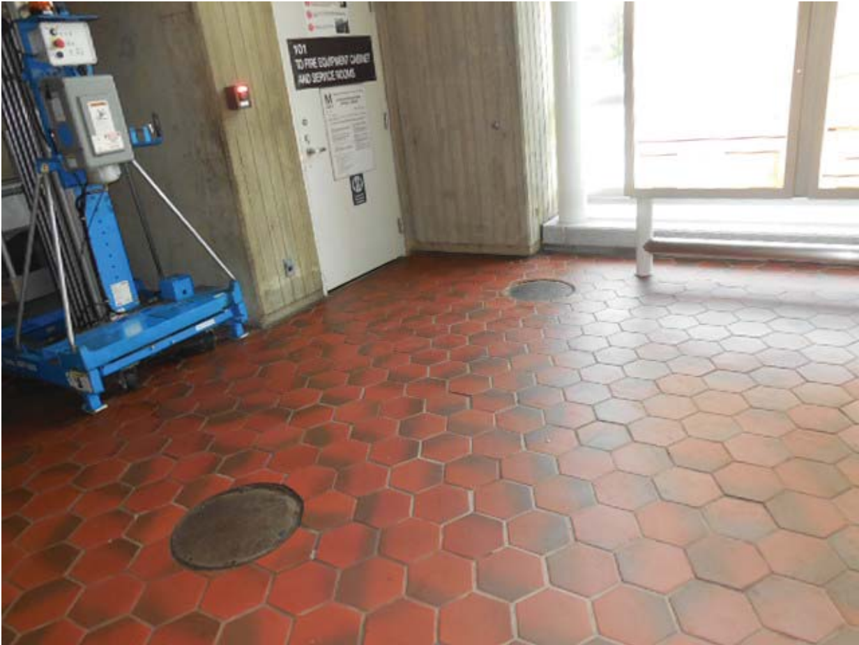
Picture 2: G05 Largo Town Center – Manholes in Mezzanine
