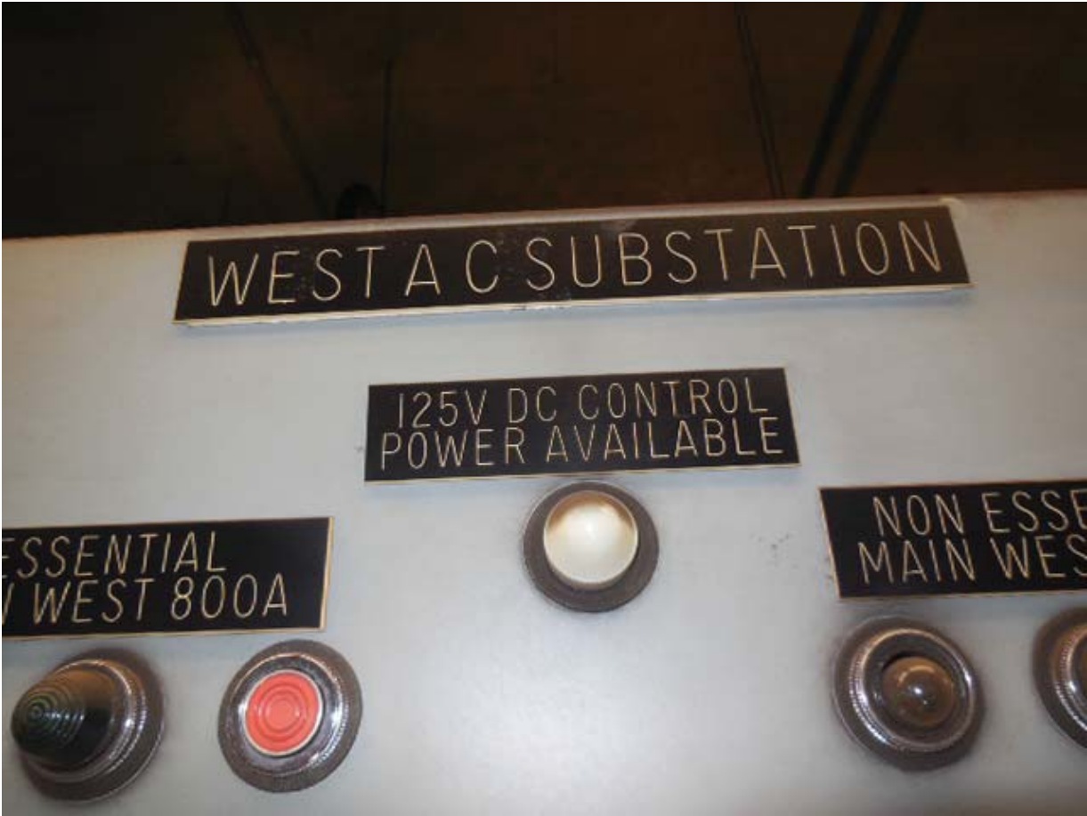
Picture 11: G01 Benning Road – West AC Substation Switchboard in Room 203
