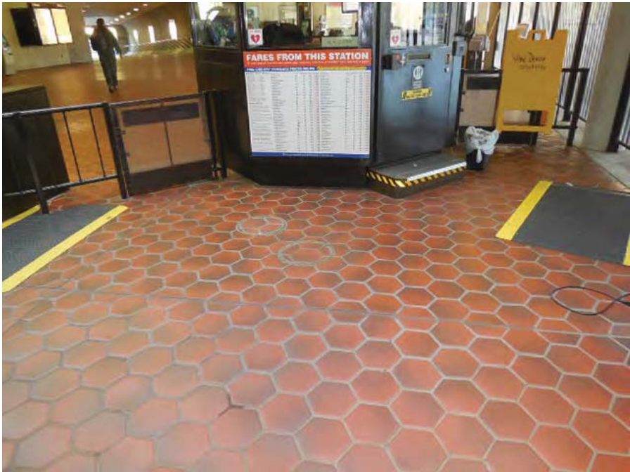
Photo #2: J03 Franconia-Springfield – Handholes near station Kiosk
