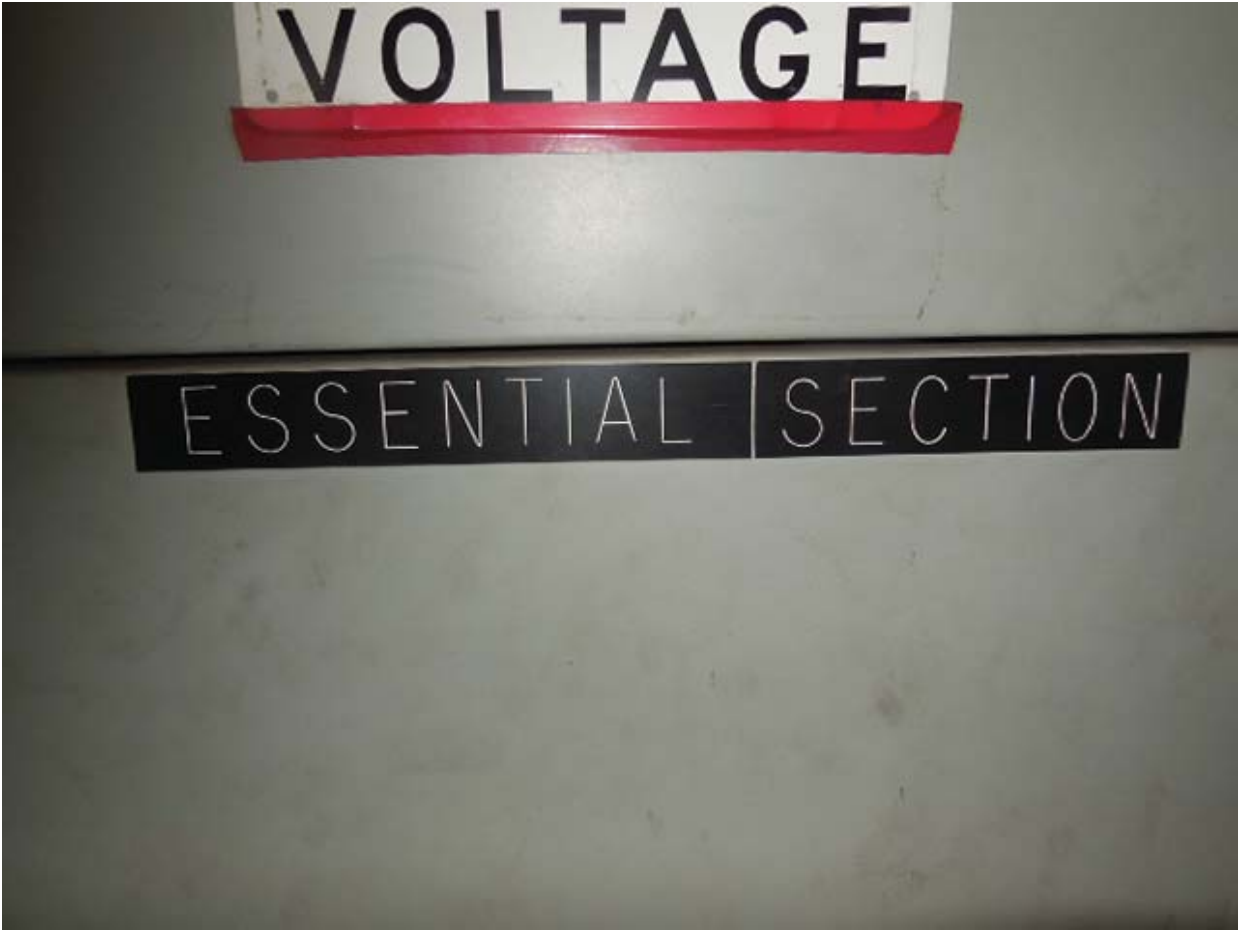
Picture 9: G03 Addison Road – Essential Section in Room 207
